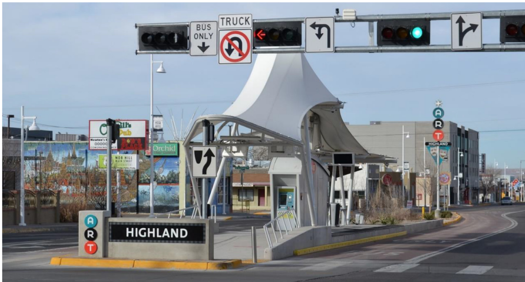
Fig. 1. A station along the Albuquerque Rapid Transit (ART) BRT line.
